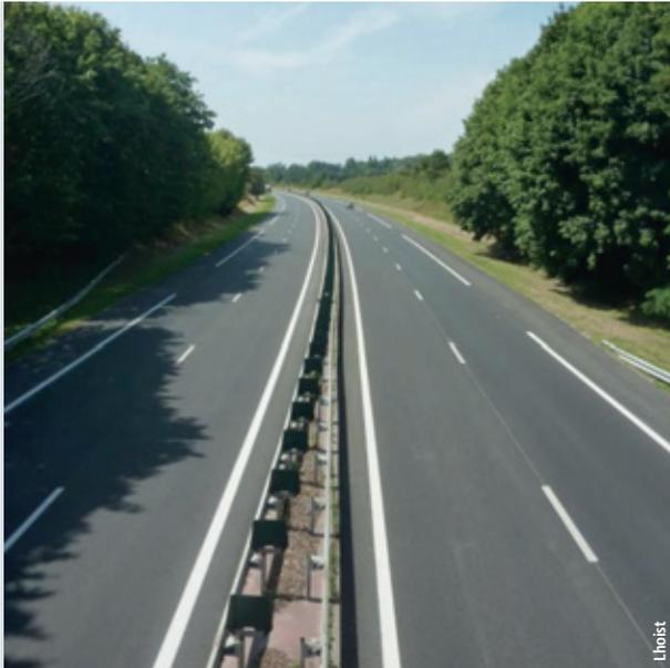
Given its impact on asphalt mixture durability, the French highway company *SANEF (Société des autoroutes du Nord et de l'Est de la France)* now requires the addition of 1.5% hydrated lime in the wearing courses of its network. Here, a A132 section near *Honfleur* in the *Calvados* department (Normandy)
