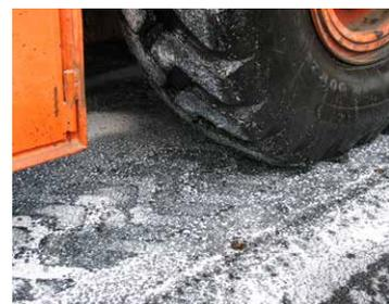
Tyres no longer stick to tack coats after spreading Asphacal® TC
